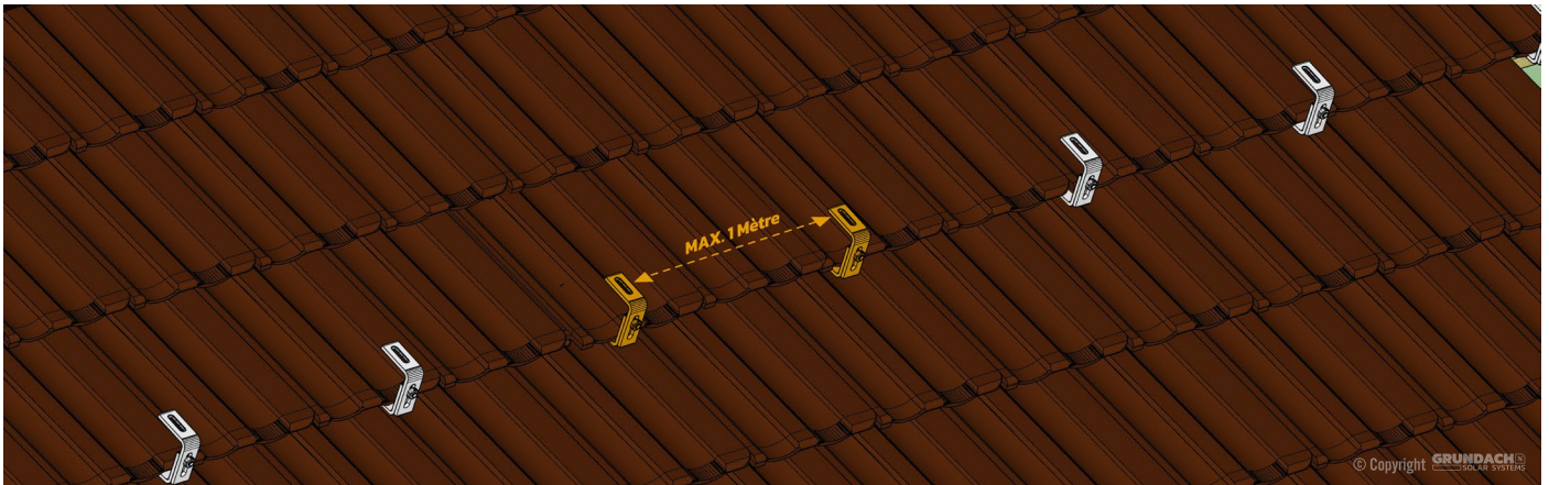
4. Positioning of the hooks on the roof. Determine the position of the hooks based on the number of panels to be installed. △ The spacing between each hook is a MAXIMUM of 1 METER.
